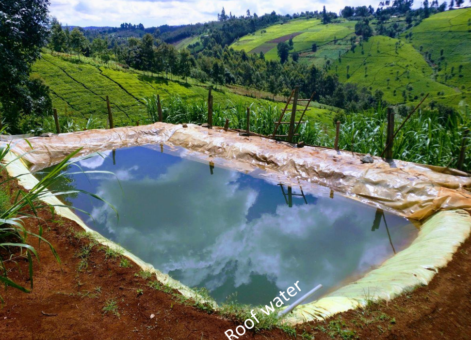
Developing water pans for runoff storage, crop irrigation
